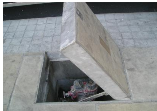
Grade 304 Stainless Steel Kent Solo Paver installed in Hemel Hempstead, London
