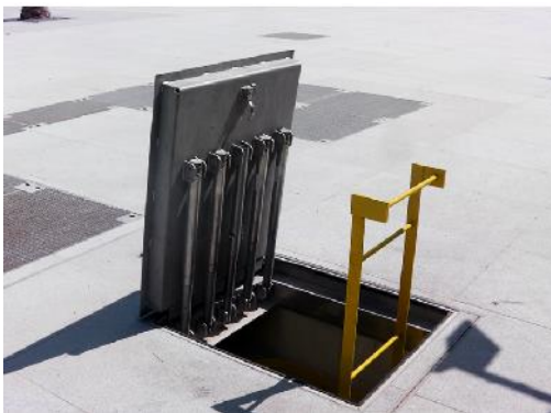
Grade 316 Stainless Steel Kent Solo Paver installed in Lusail, Qatar
